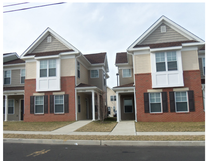
Centerville South Housing in Camden, NJ
